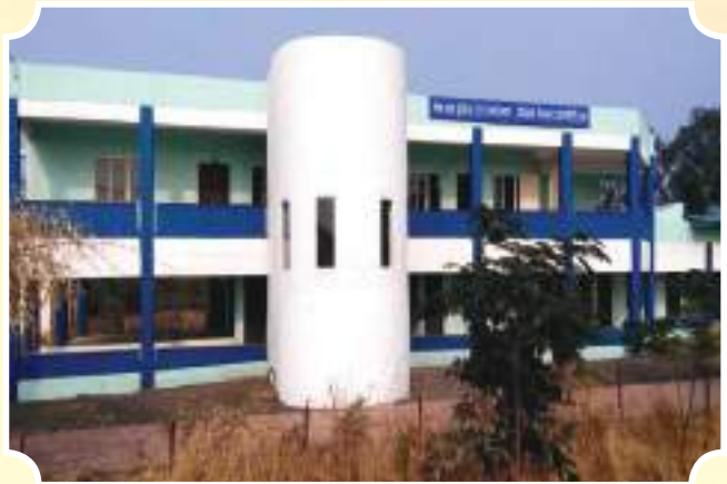
RSETI DHAR BUILDING
